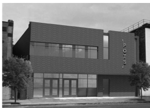
After POTS renovation.
