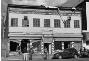
POTS before renovation.
