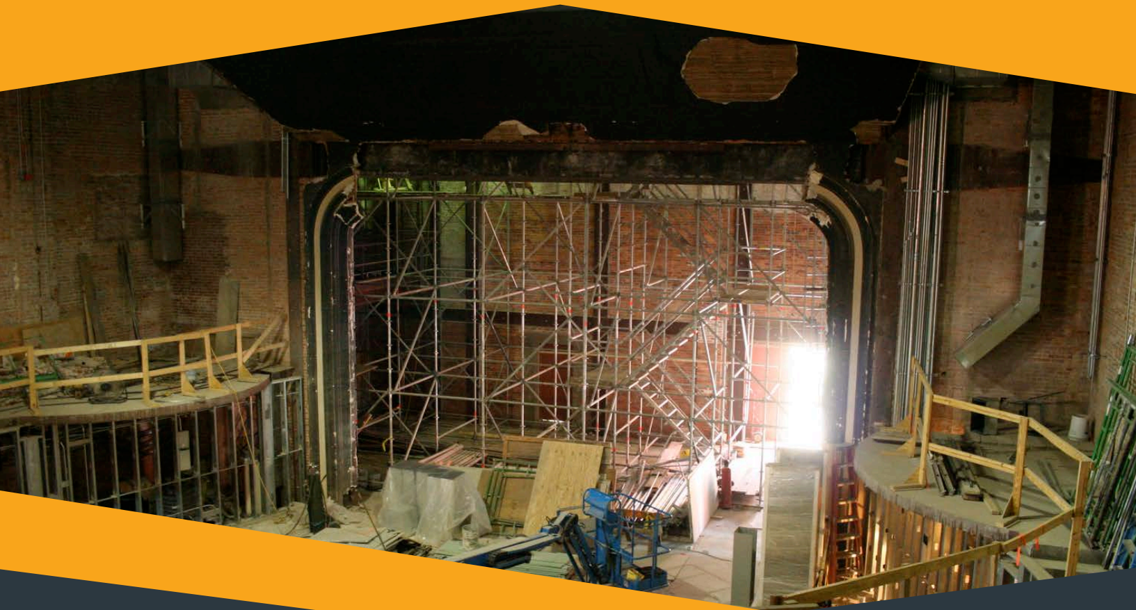
Above: Restoration efforts underway for the Athens Theater
