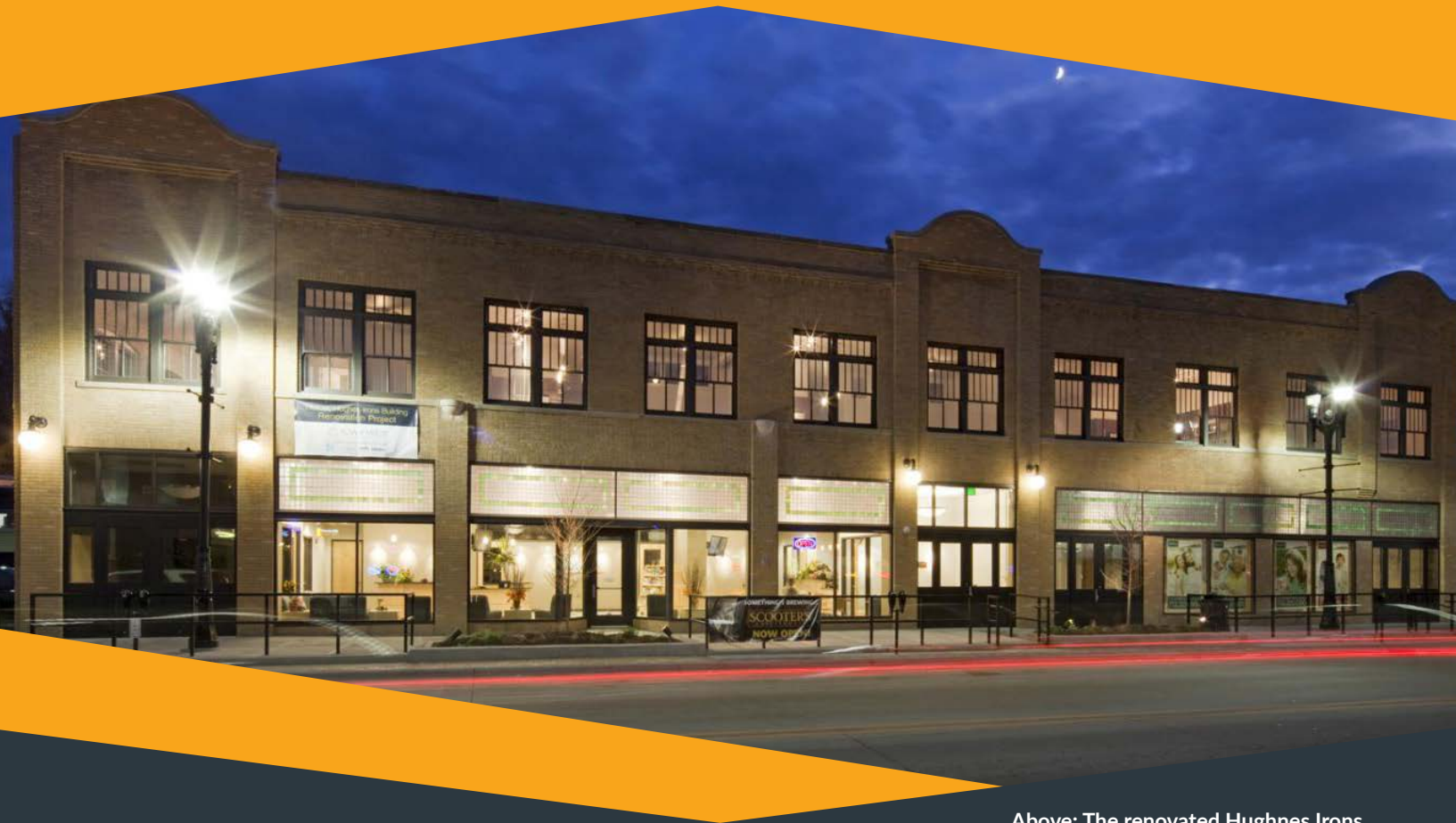
Above: The renovated Hughnes Irons Building
