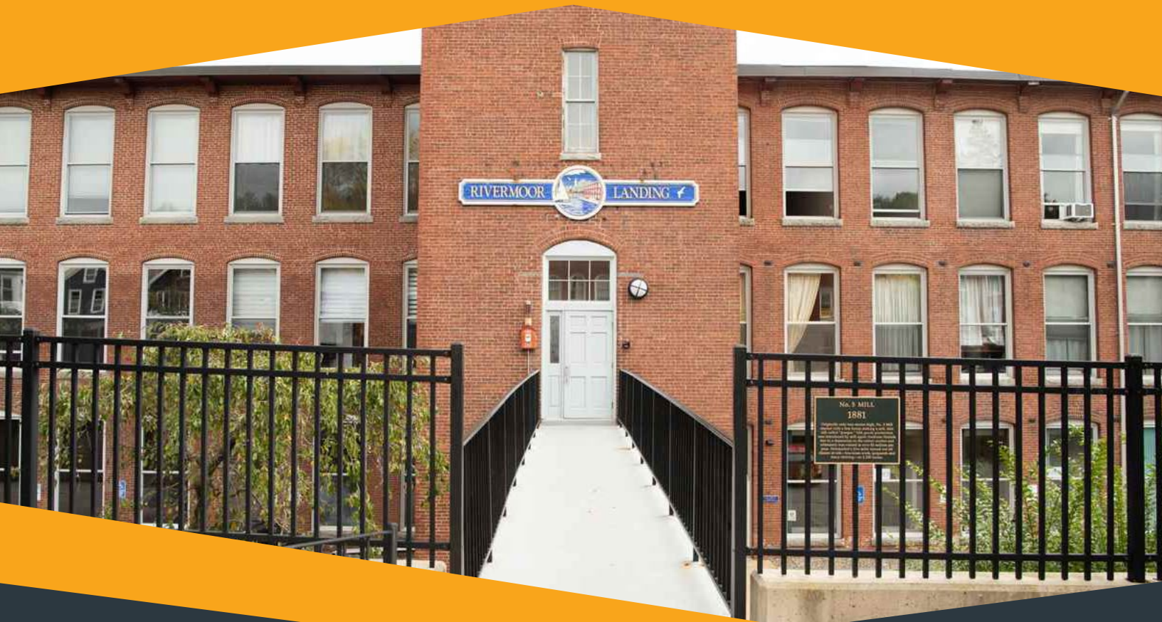
Above: A renovated building along the river in Newmarket, NH.
