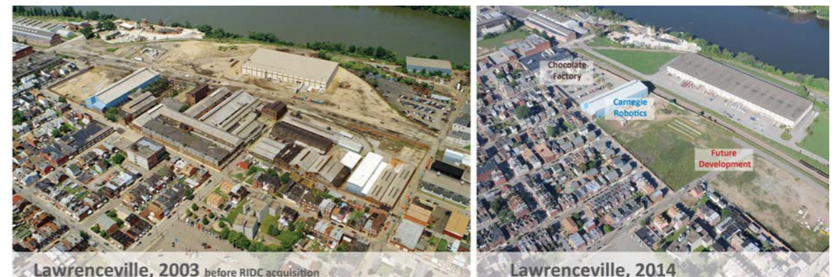
Lawrenceville, 2003 before RIDC acquisition
