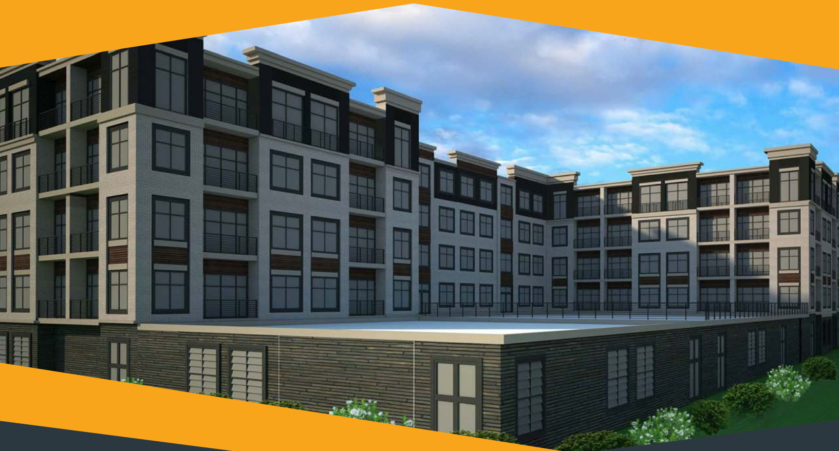
Above: The Station at Grant Avenue, a mixed-use redevelopment project in Plainfield on the edge of the 7th district.
