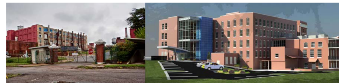
Dan River Inc. Rehabilitation Danville, VA
