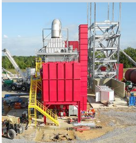
Top: Construction of Westervelt Pellet I, Inc. is underway
