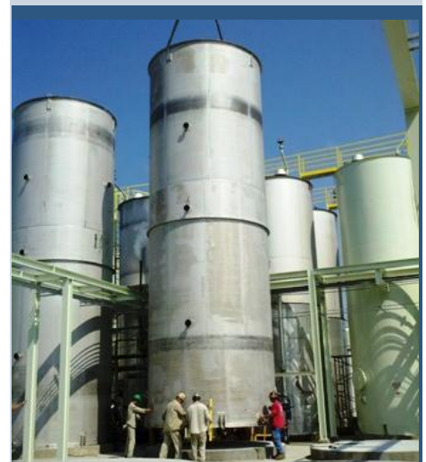
Top: Resinall Corps' manufacturing facility in Hattiesburg, MS
