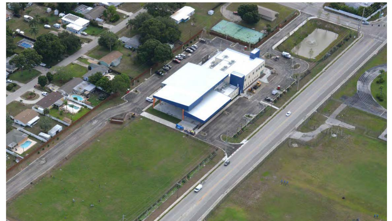
Above: A July 2019 view from overhead and the front of the nearly completed facility
