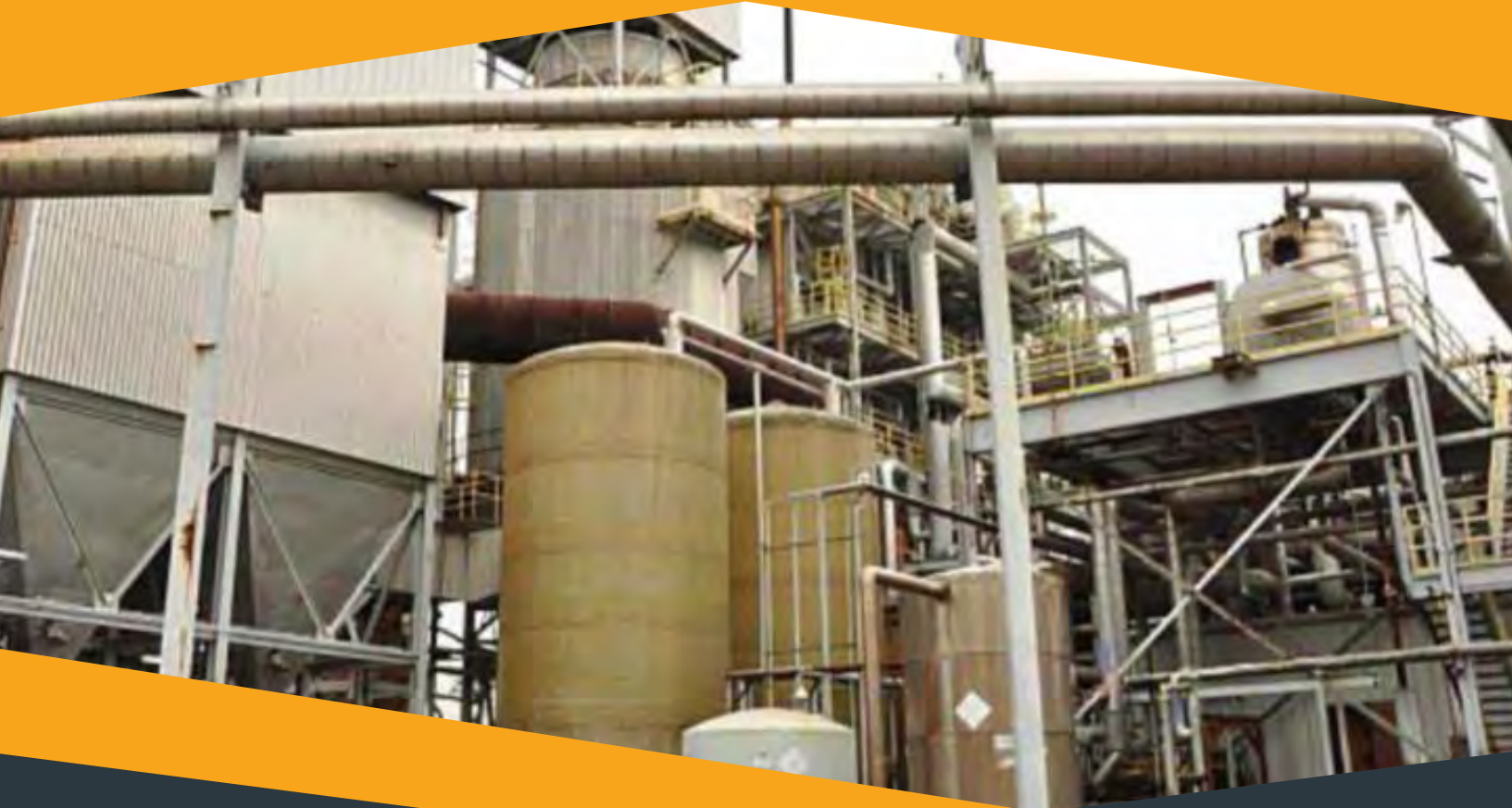
Above: The retooled former coal plant in Thomaston, GA
