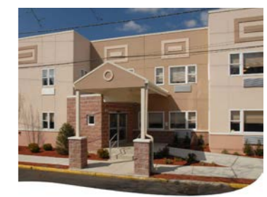
Doctors Subacute Care Paterson, NJ Healthcare facilities make up more than 10% of NMTC projects nationwide. The NMTC financed Doctors Subacute Care, a residential care facility in Paterson.
