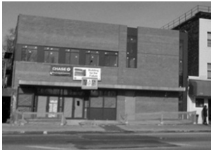
POTS during renovation.
