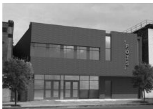
After POTS renovation.
