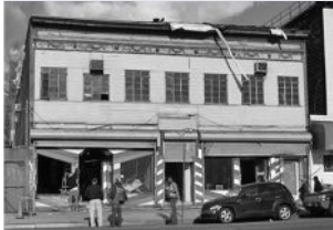
POTS before renovation.
