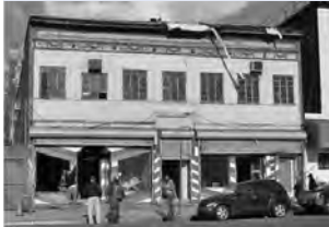
POTS before renovation.
