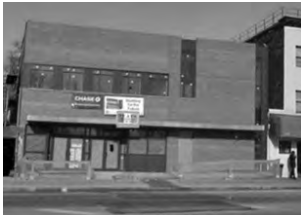
POTS during renovation.
