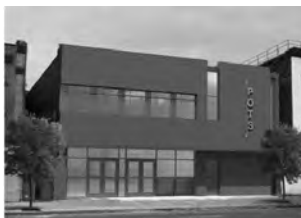
After POTS renovation.
