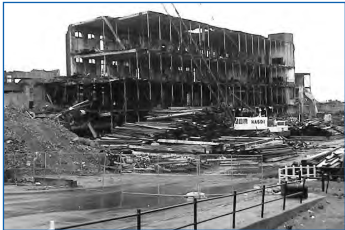
During the construction.
