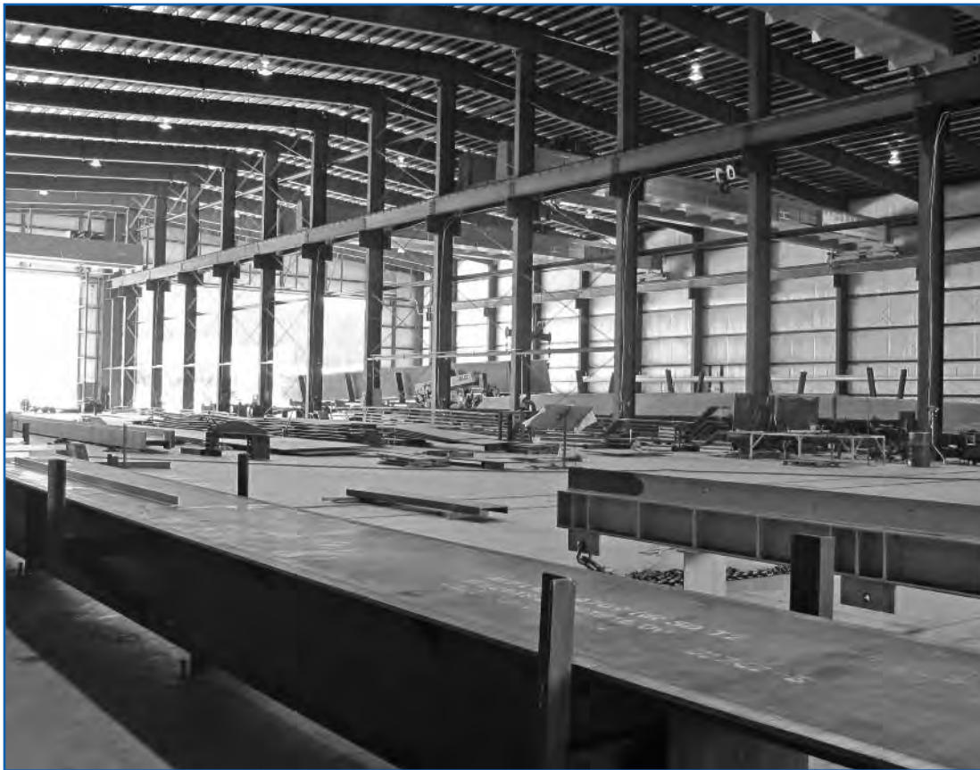
Stinger Welding interior
