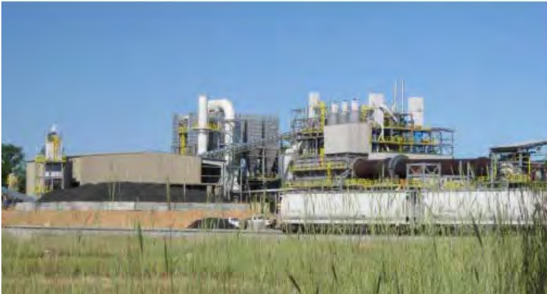
Construction of a new manufacturing facility in Barnwell, South Carolina created 499 construction jobs and 116 new direct jobs. Photo from the NMTC Coalition’s “NMTC At Work” report (Dec. 2012).
