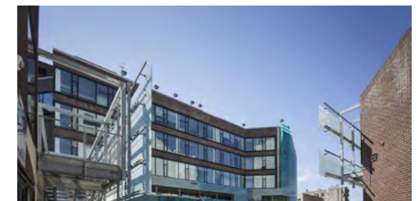
BEDFORD STUYVESANT RESTORATION PLAZA Brooklyn, NY
