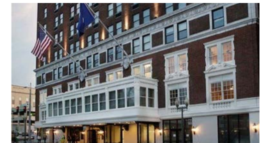
Rehabilitation of the Patrick Henry Hotel Roanoke, VA
