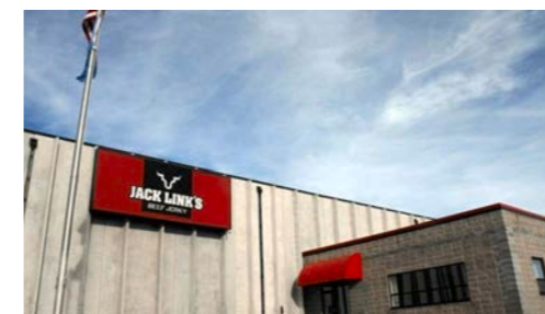
Jacks Links Beef Jerky Manufacturing Plant Alpena, SD
